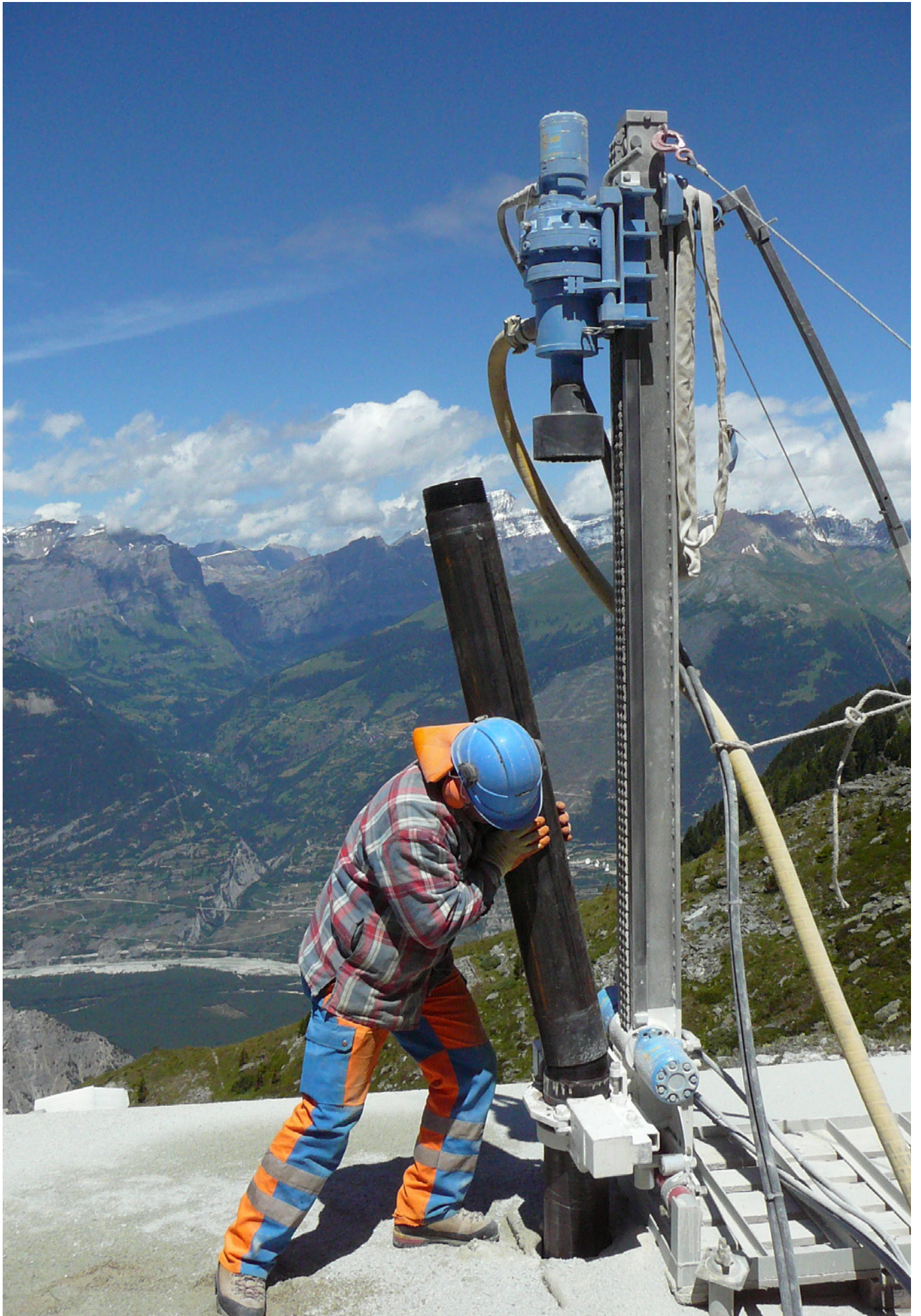
Mounty® H 92 S, diameter 216 mm, length 40 m, test drilling by the dam Illsee, Leuk, Switzerland
